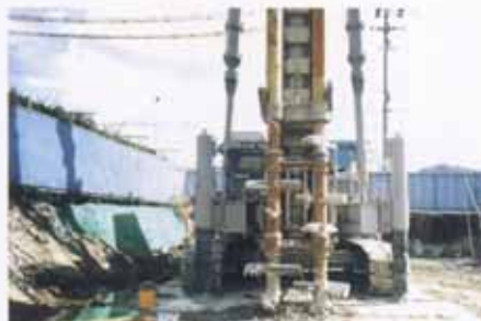
Work in Progress (on Land)
